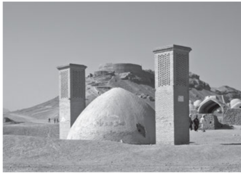
Natural ventilation, wind towers and yakchal or ice storage, Yazd, Iran
